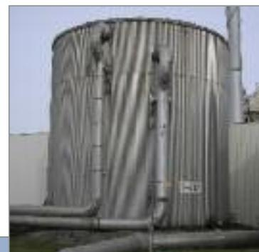
the building of the water-purification plant. Here the surface water is pumped by high-pressure pumps to six double-layer pressure filters. The pressure filters remove the particles: manganese and iron from the surface water. By reducing the acidity, the carbonates are converted into carbon dioxide, which is removed in a decarbonisation unit.
